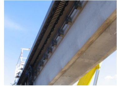
Hybrid/High Speed Hybrid LSM on Guideway
